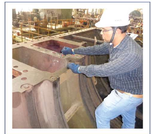
Visual Inspection of LP Casing
