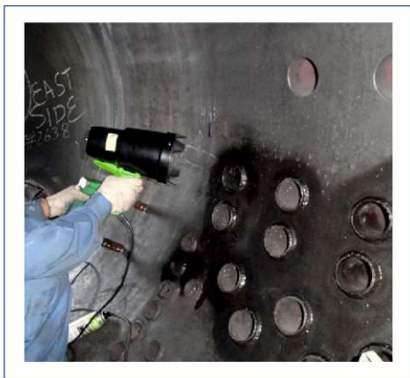
Magnetic Particle Inspection of Boiler Drum
