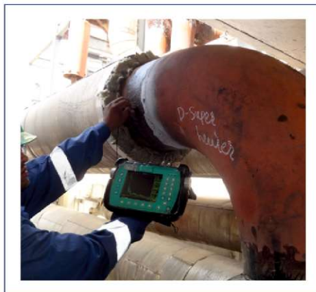
Ultrasonic Testing of De SuperHeater Pipe
