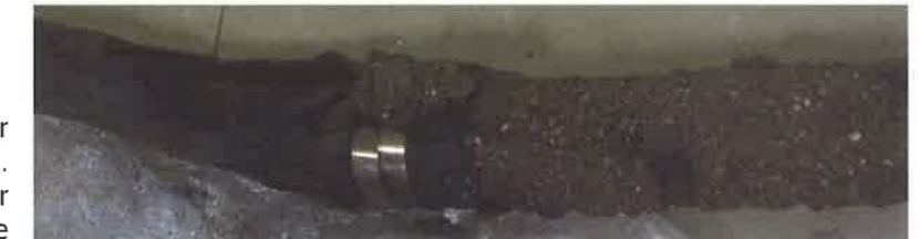
Figure 4: Connection of the earthing continuity wires with aluminium sheath.
